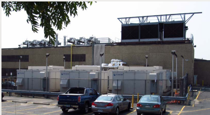
Fuel cell-based microgrid in Garden City, NY after Hurricane Irene
