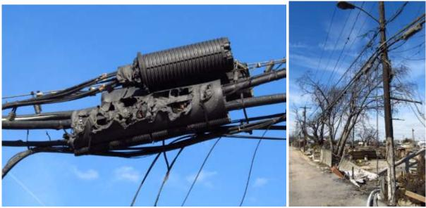
Fig. 33. Damage from a fire affecting communications infrastructure.
