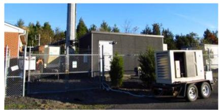
Fig. 21 A cell site with multiple genset (3 portable and one permanent) at the intersection of I 95 and I 195 in New Jersey.
