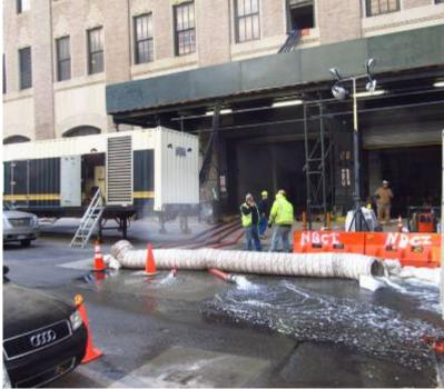
Fig. 3. Water being pumped out and a diesel generator running at the entrance on Barclay Street for Verizon's main central office in Manhattan.
