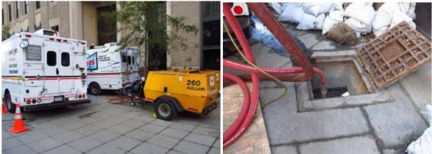
Fig. 6. Emergency cable pressurization units at 140 West Street. The image on the right shows the pressurized air injection nozzle.
