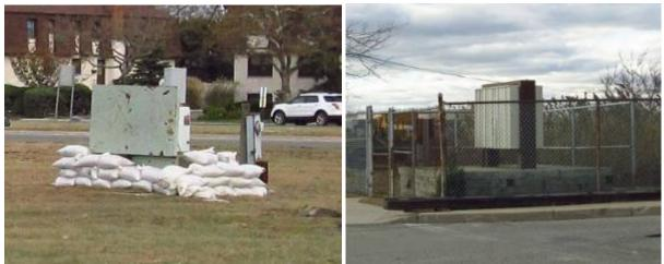
Fig. 32. A vault (left) and a DLC RT cabinet (right) in the Rockaway Peninsula.
