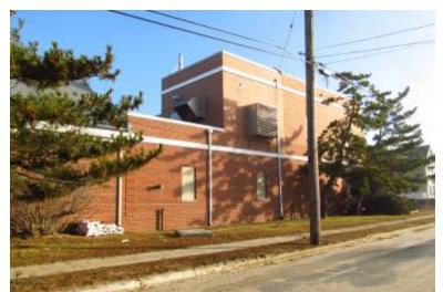
Fig. 12. Verizon's central office in Lavallatte. Notice the genset located on the second floor.
