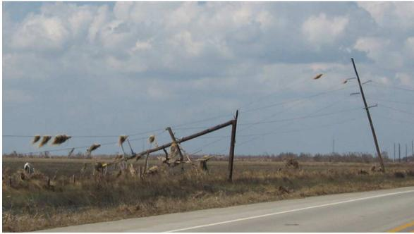
Fig. 3. Broken and tilted poles caused by Hurricane Ike in the only line serving the Bolivar Peninsula area.
