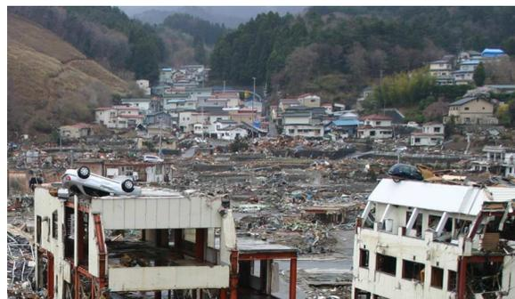
Fig. 2. Onagawa, Japan. While all buildings and infrastructure in the foreground were demolished by the tsunami, there is little damage in the background area higher on the hills where the tsunami did not reach.
