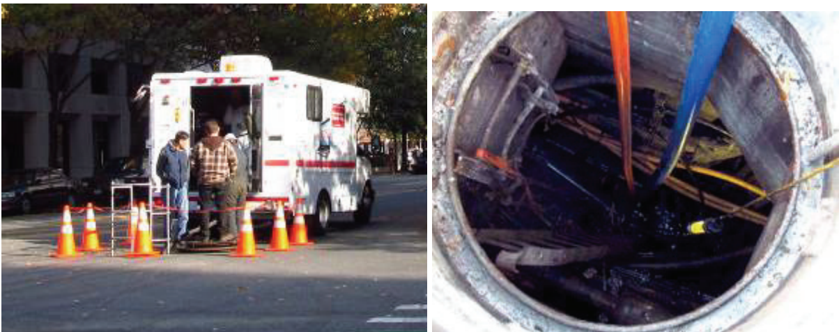
Fig. 24. Left: A Verizon's truck working next to manhole. Right: A manhole still with water.
