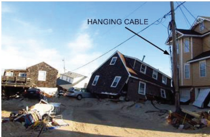
Fig. 25. A severed telecom cable hanging from the pole on the right.
