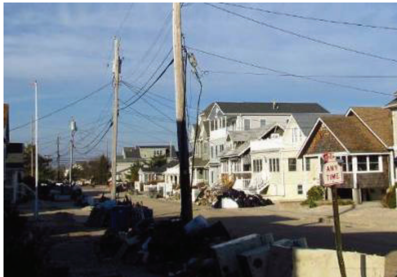
Fig. 26. Damage to the pole nearest the sea in Ortley Beach
