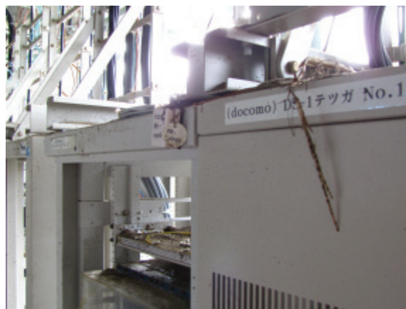
Fig. 45. NTT Docomo (wireless) switching equipment at NTT East's (wire-line) Nobiru CO.
