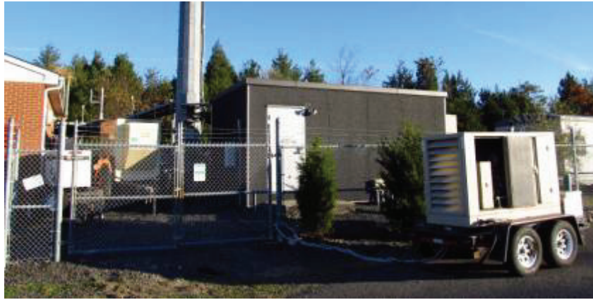
Fig. 33 A cell site with multiple genset (3 portable and one permanent) at the intersection of I-95 and I-195 in New Jersey after superstorm Sandy.
