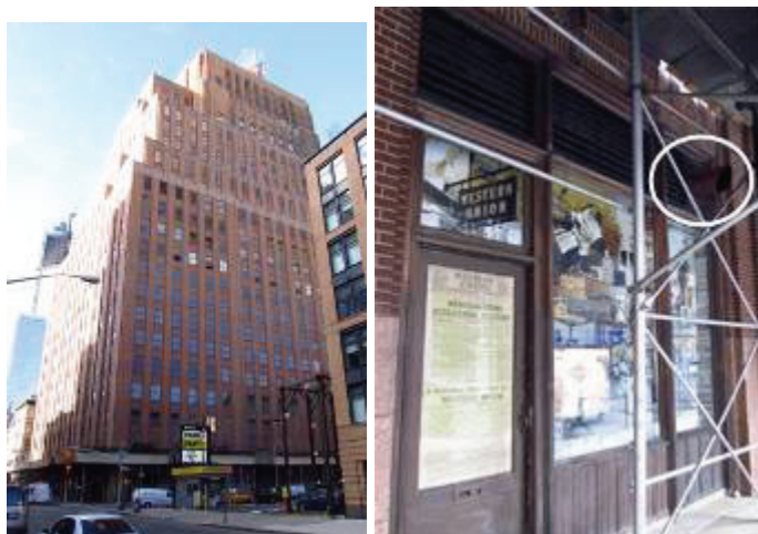
Fig. 53. Data center at 60 Hudson Street. Notice the diesel generator exhaust on the photo on the right.
