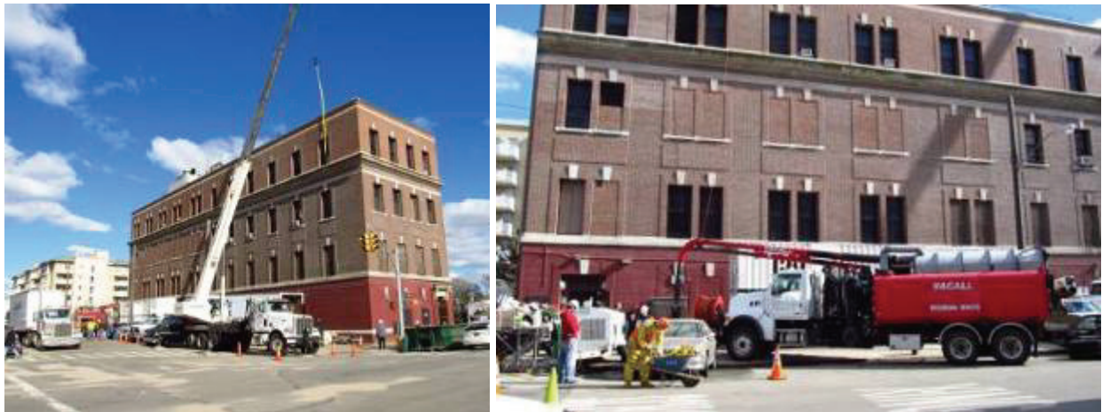
Fig. 16. Verizon's central office at Rockaway Beach. The photo on the right shows a large portable genset behind the waste liquids vacuum pump.
