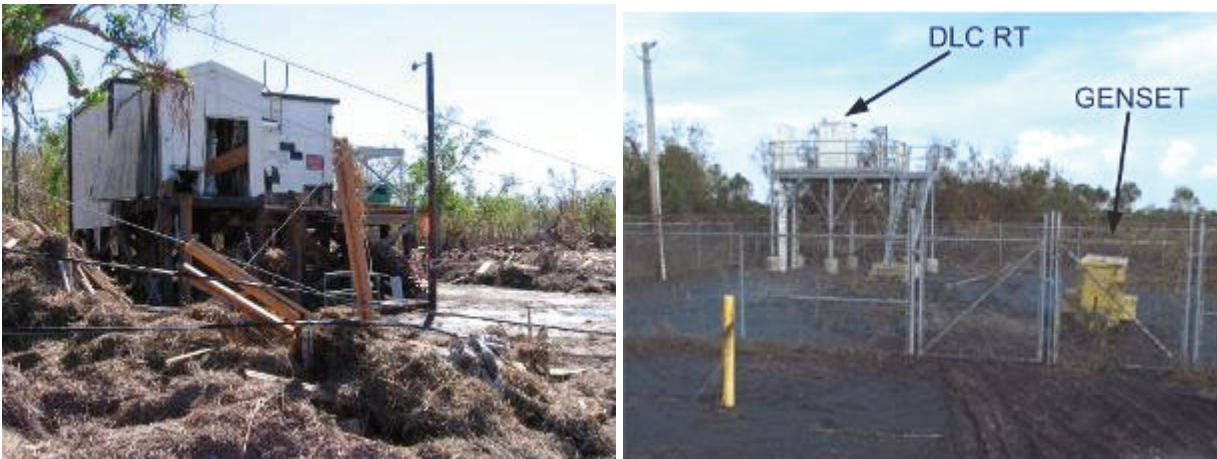
Fig. 8. Left: Remains of Delacroix CO after Hurricane Katrina. Right: Same site after Hurricane Isaac. Notice the yellow portable genset deployed to power the RT on the platform.
