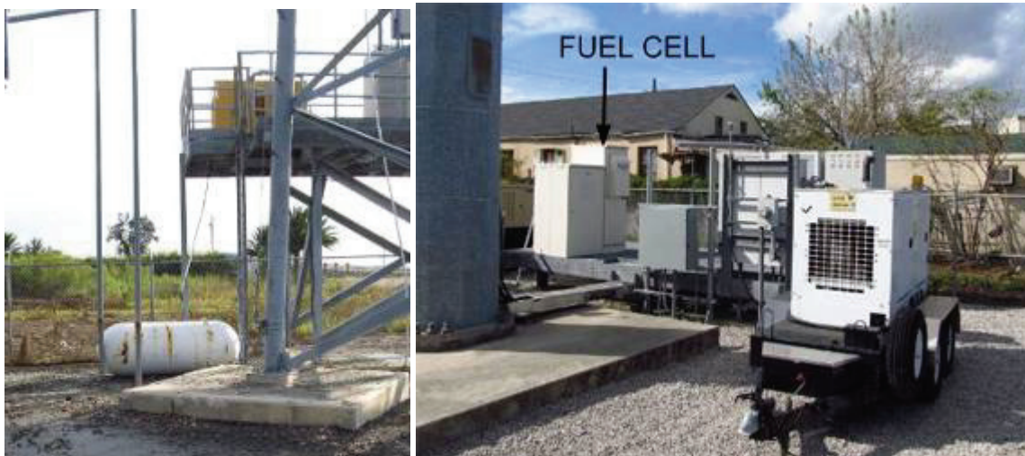
Fig. 35. Power backup alternatives for cell sites in the aftermath of Hurricane Isaac. Left: Propane tank damage by Isaac's storm surge. Right: Fuel cells.
