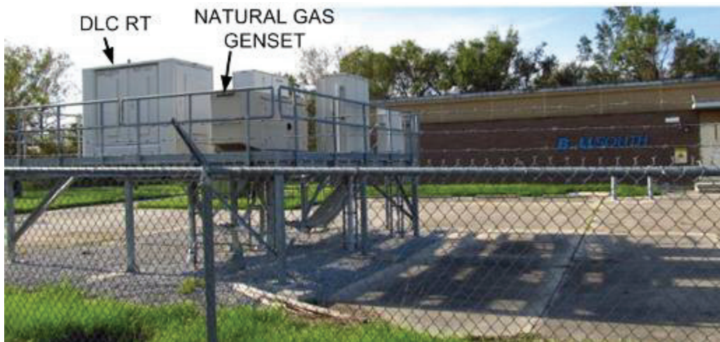
Fig. 9. In the background the building of Bellsouth's former St. Bernard CO flooded by Katrina. Equipment inside this building was never replaced and parts of its functions were restored with the DLC RT shown in the foreground and installed after Katrina.
