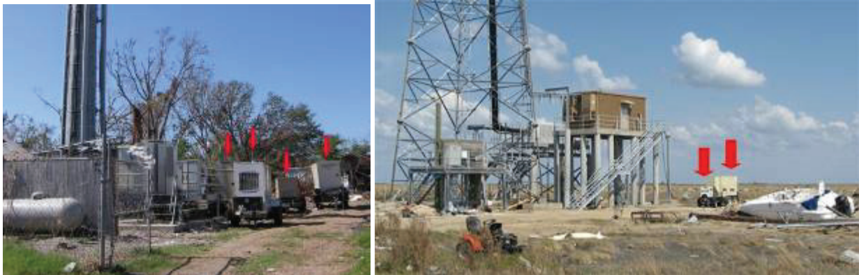
Fig. 32. Multiple portable gensets deployed to cell sites in the aftermath of hurricanes. Left: Katrina. Right: Ike.
