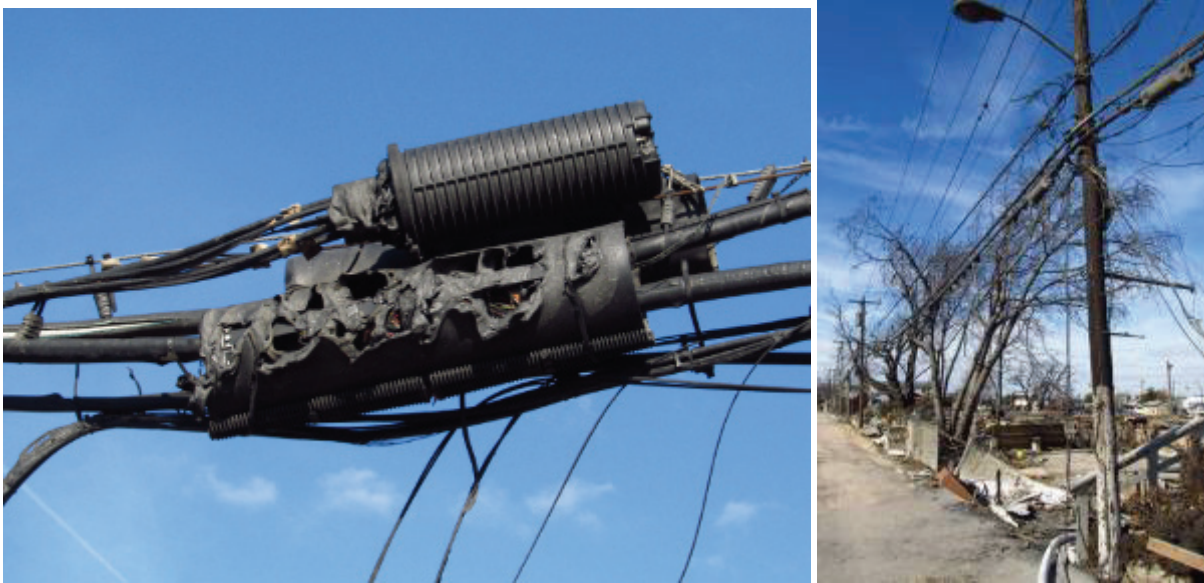
Fig. 23. Damage from a fire affecting communications infrastructure.
