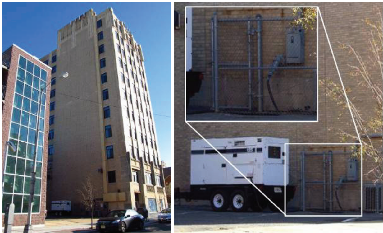
Fig. 29 A rooftop cell site in Ausbury Park powered by a genset at street level. Notice the standard connector for the genset.
