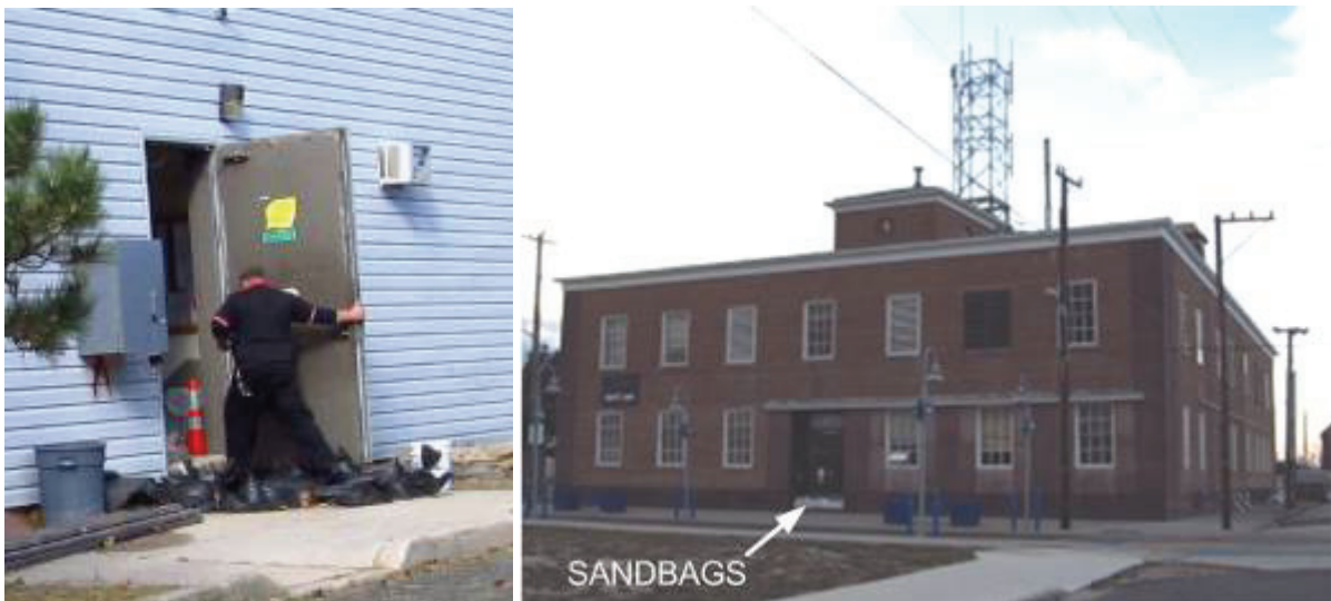
Fig. 21. Verizon's central offices in Brigantine (Left) and Wildwood (Right). Notice in both cases the sandbags at the doors.
