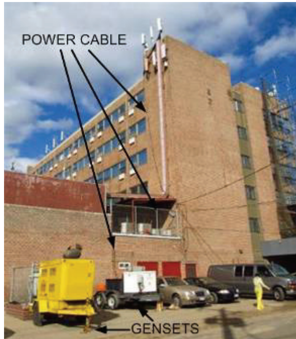
Fig. 30. A rooftop cell site in the Rockaway Peninsula.
