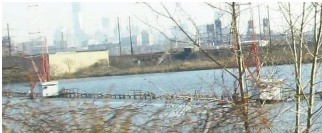
Fig. 55. Transmission towers for WEPN, damaged by Sandy.
