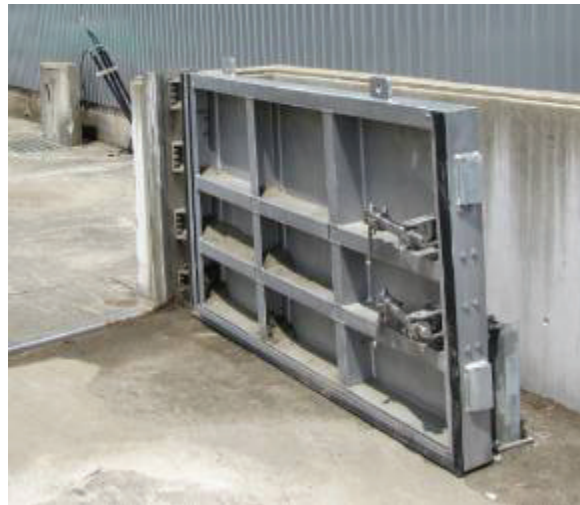
Fig. 20. Flood gate in Unosumai central office, Japan.
