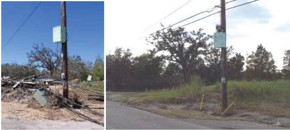
Fig. 50. Left: A pole mounted CATV amplifier and power supplier with a pad mounted natural generator destroyed by Katrina's storm surge. Right: The same CATV equipment after Isaac powered by a camping portable genset placed on top of the CATV amplifier and power supply
