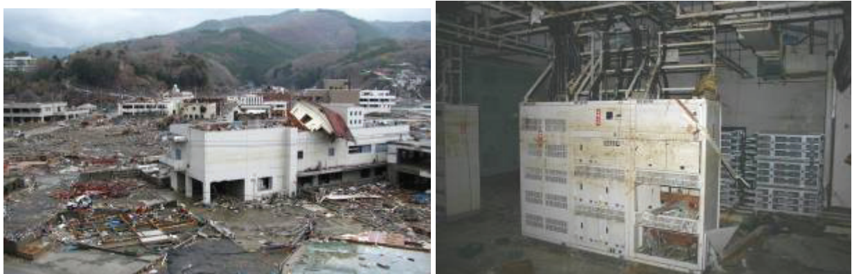
Fig. 18. Onagawa CO Building. Left: Exterior. Right: Interior; power room.
