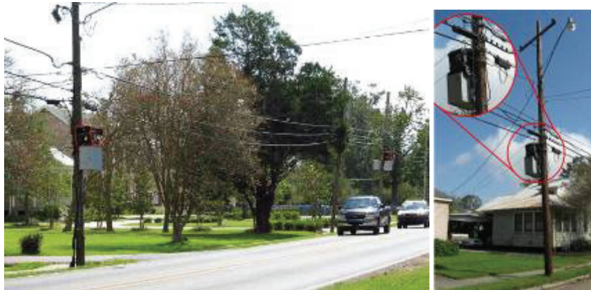
Fig. 51. Examples of camping-type portable gensets used to power CATV pole mounted equipment. Left: After Isaac. Right: After Gustav.
