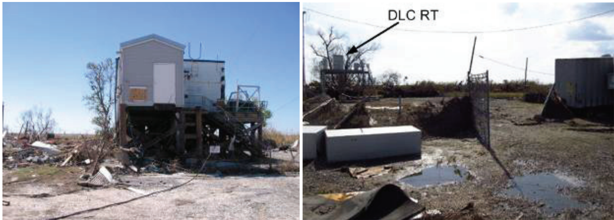
Fig. 7. Left: Remains of Yscloskey CO after Hurricane Katrina. Right: Same site after Hurricane Isaac
