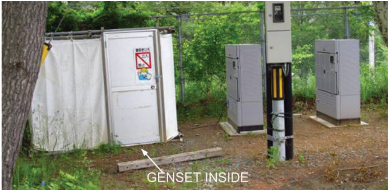
Fig. 10. Two DLC RTs uses to partially restore service in the area of NTT's Onagawa CO that was submerged by the tsunami.
