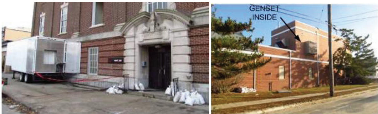
Fig. 17. Left: Verizon's central office in Long Beach. Right: Verizon's central office in Lavallatte. Notice the genset located on the second floor.
