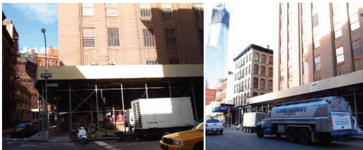
Fig. 54. Two views of the 60 Hudson Street data center showing additional small gensets in the area and a truck with diesel to replenish the fuel tanks at this site.
