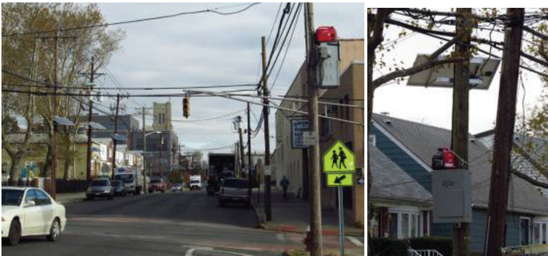
Fig. 48. CATV equipment in Bayonne, NJ.
