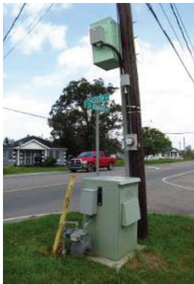
Fig. 49. A pad mounted natural gas generator powering CATV equipment after Hurricane Isaac.
