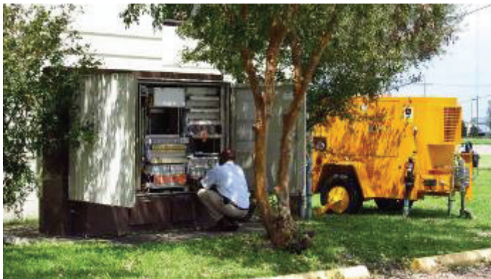
Fig. 12. Portable gensets deployed to power DLC RT after Isaac. The photo on the right shows both a pre-Katrina RT at ground level and a post-Katrina RT on a platform with a natural gas generator. It is unknown why a portable diesel genset was deployed at this site.
