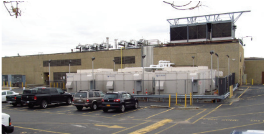
Fig. 22. Fuel cells at Verizon's central office in Garden City.
