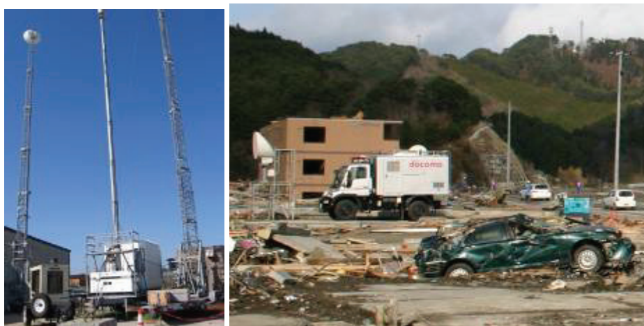
Fig. 43. Microwave repeater units linking cell sites. Left: in Biloxi, MS after Katrina. Right: in Otsuchi, Japan, after the March 2011 tsunami.
