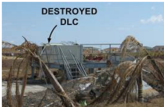
Fig. 11. DLC RT destroyed by Hurricane Ike. The one on the right had been installed after Hurricane Rita in order to partially restore service lost when Sabine Pass' CO was destroyed.
