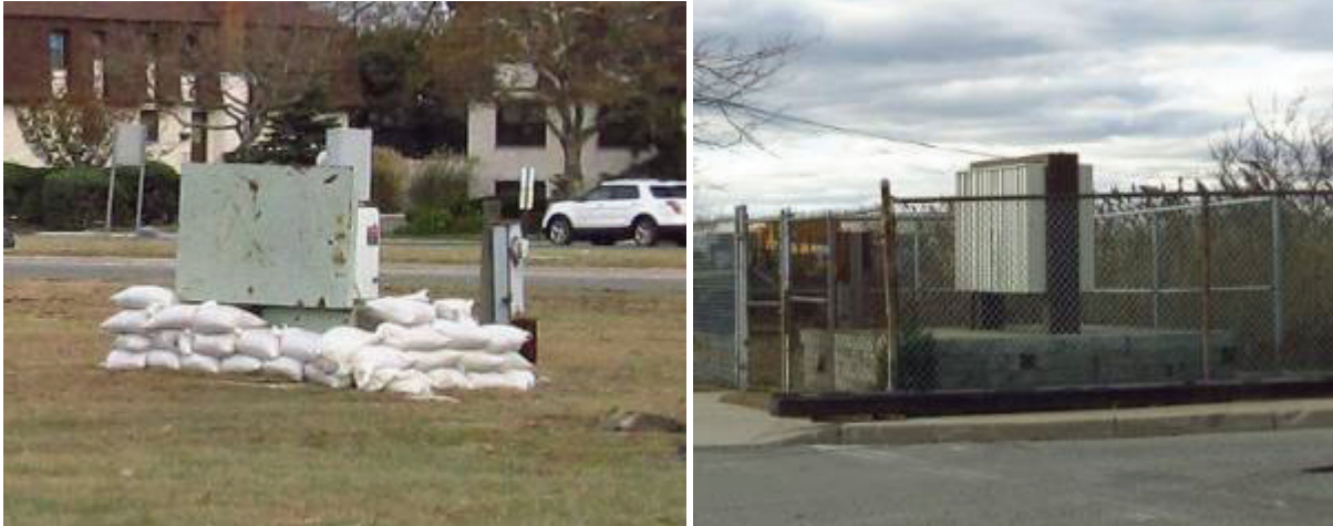
Fig. 13. A vault (left) and a DLC RT cabinet (right) in the Rockaway Peninsula.
