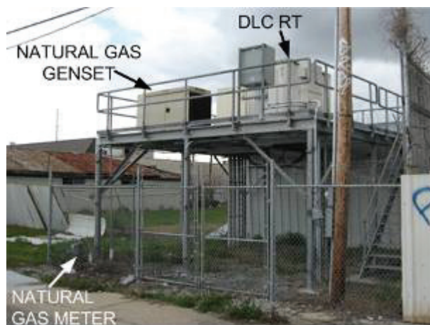
Fig. 6. A DLC RT in New Orleans installed a few months after Hurricane Katrina. Notice the natural gas generator.
