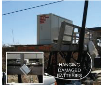
Fig. 11. DLC RT destroyed by Hurricane Ike. The one on the right had been installed after Hurricane Rita in order to partially restore service lost when Sabine Pass' CO was destroyed.
