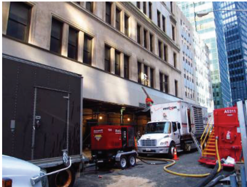
Fig. 14 Pearl Street side of Verizon's central office at 104 Broad Street.
