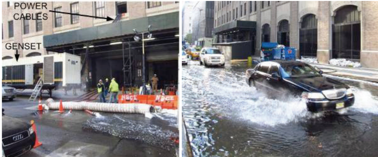
Fig. 4. Right: Water being pumped out and a diesel generator running at the entrance on Barclay Street for Verizon's main central office in Manhattan. Left: Flooding on Barclay St. from water being pump out of Verizon's central office at 140 West Street.
