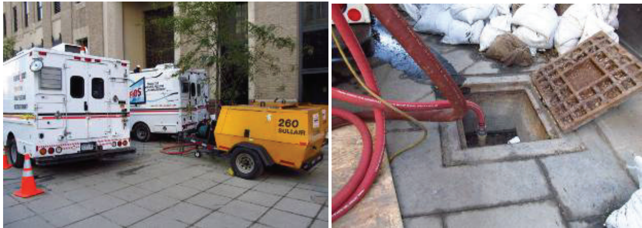
Fig. 5. Emergency cable pressurization units at 140 West Street. The image on the right shows the pressurized air injection nozzle.
