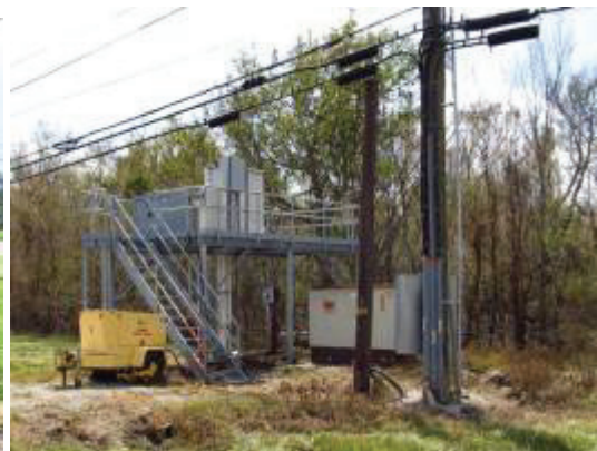
Fig. 12. Portable gensets deployed to power DLC RT after Isaac. The photo on the right shows both a pre-Katrina RT at ground level and a post-Katrina RT on a platform with a natural gas generator. It is unknown why a portable diesel genset was deployed at this site.
