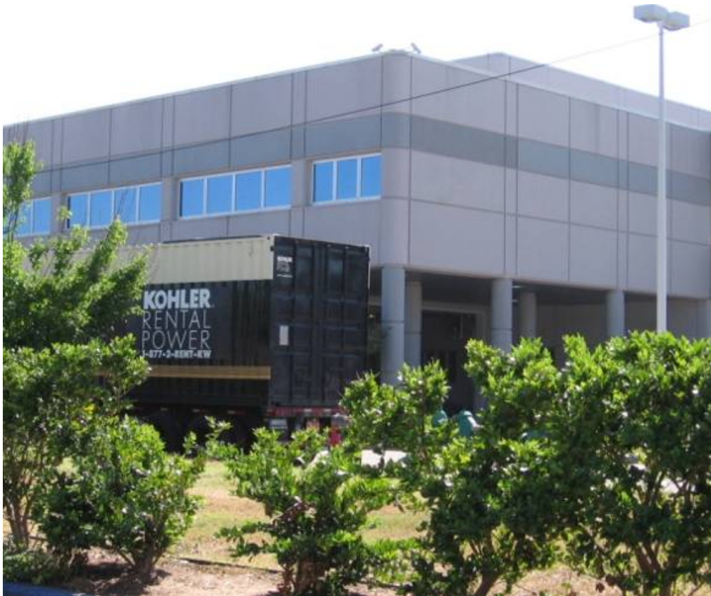
Fig. 9.5. Public safety building in Biloxi, MS
