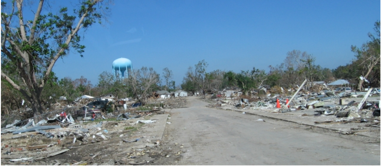
Fig. 3.2. Total destruction in Biloxi, MS
