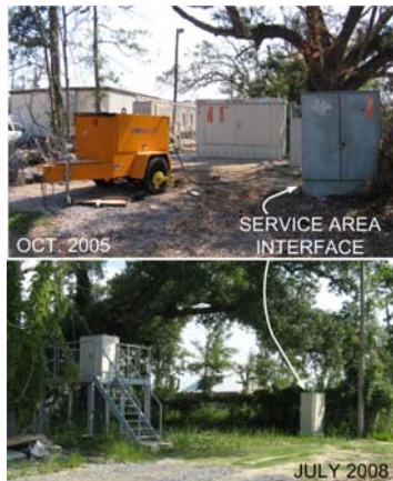
Figure 13 The same DLC site in Waveland, MS.
