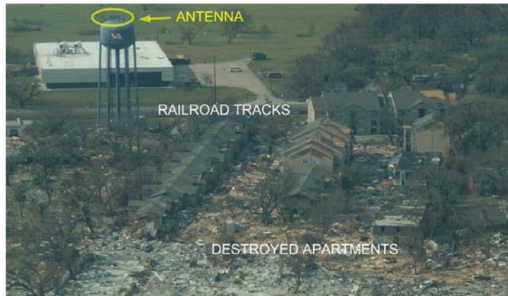
Fig. 6.20. Cell site located east of Gulfport that uses a water tank as tower [7]
