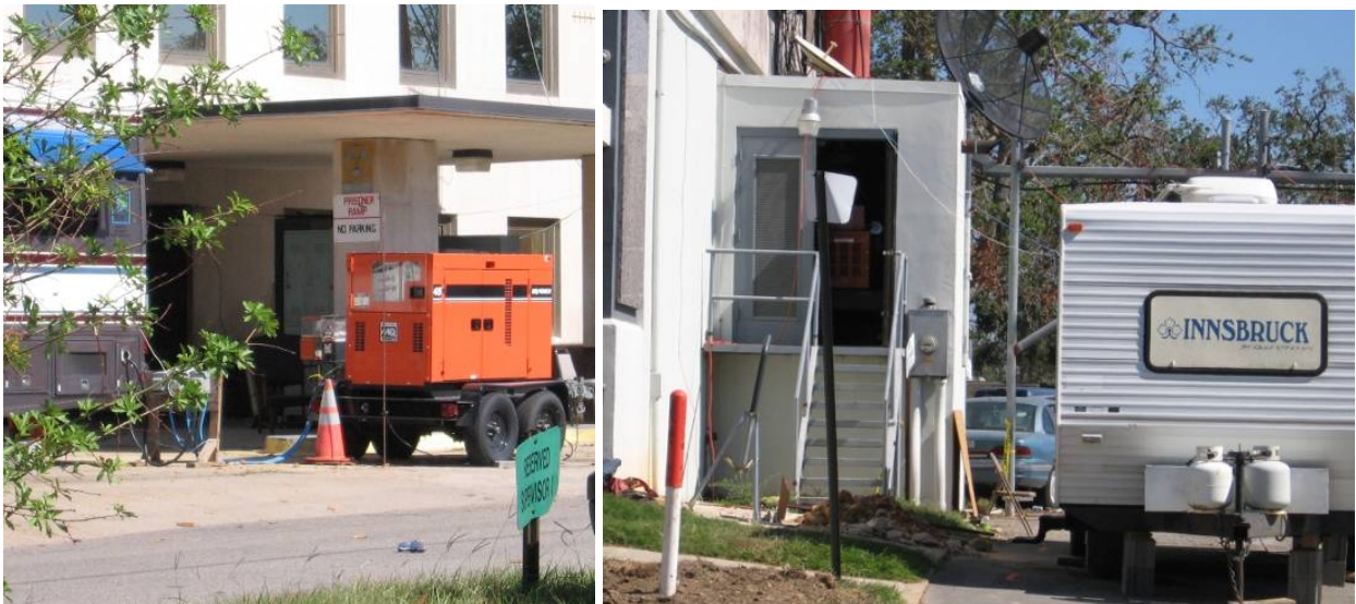
Fig. 9.4. Jackson County Emergency Operation Center in Pascagoula, MS
