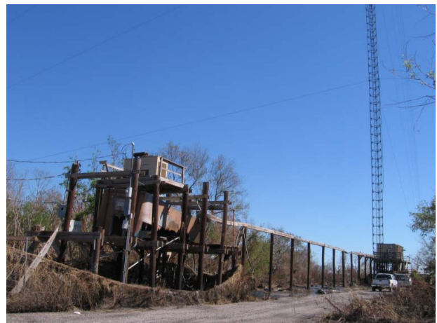
Fig. 16. KQLD-FM Radio transmitter and tower in Delacroix, LA. A genset is on top of the damaged structure on the left.
