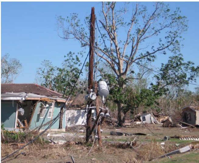
Fig. 4. Damage to the electric distribution grid near Pt. A La Hache, LA.
