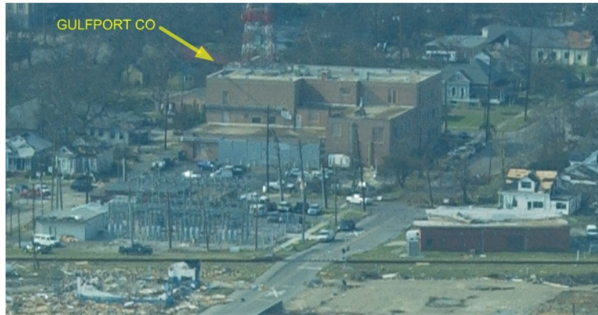
Fig. 5.22. Gulfport CO on August 31 or September 1, 2005 [7]
