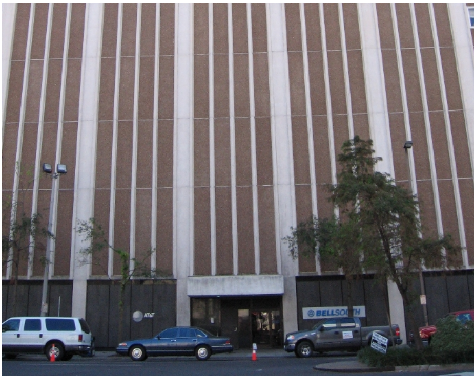
Fig. 5.11. New Orleans Main CO entrance
