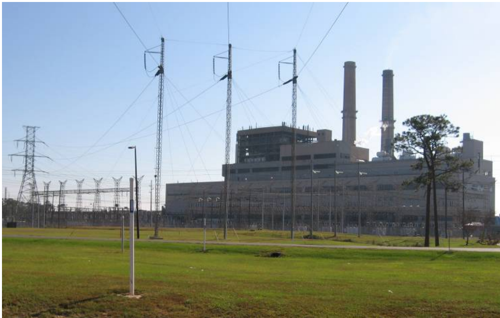
Fig. 8.1. Mississippi Power, Watson Electric Generating Plant
