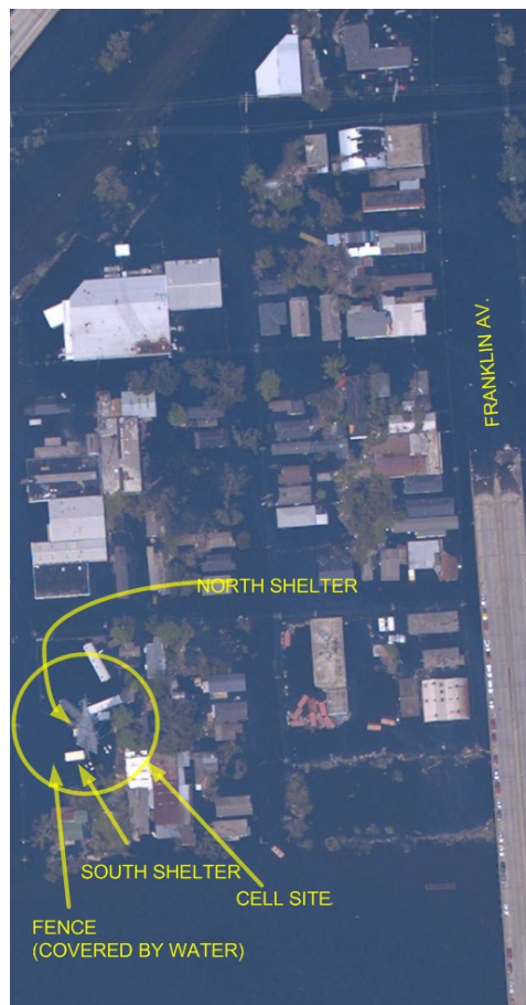
Fig. 6.52. Aerial picture of cell site northeast of downtown New Orleans, August 31, 2005 [6]
