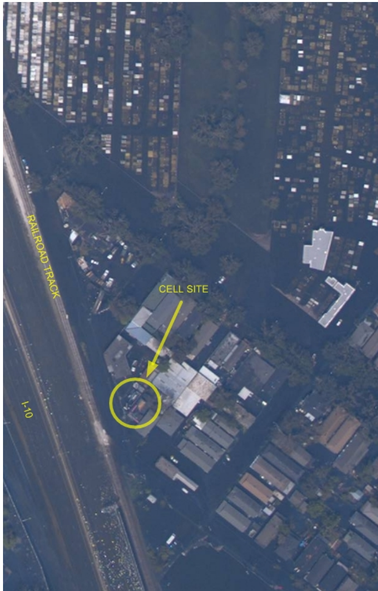
Fig. 6.48. Aerial picture of a site northeast of downtown New Orleans
