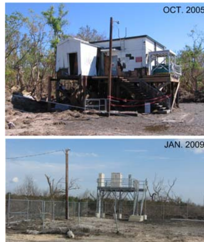
Figure 10 Delacroix central office site just after Hurricane Katrina and approximately 3 years later.
