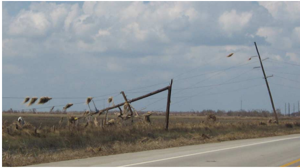
Fig. 3. Broken and tilted poles caused by Hurricane Ike in the only line serving the Bolivar Peninsula area.
