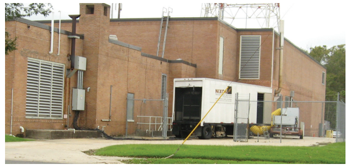
Fig. 3. A large portable generator outside Goodwood central office in Baton Rouge, Louisiana, less than a week after Hurricane Gustav.
