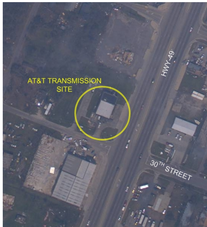
Fig. 5.80. Aerial view of AT&T site, September 4, 2005 [6]
