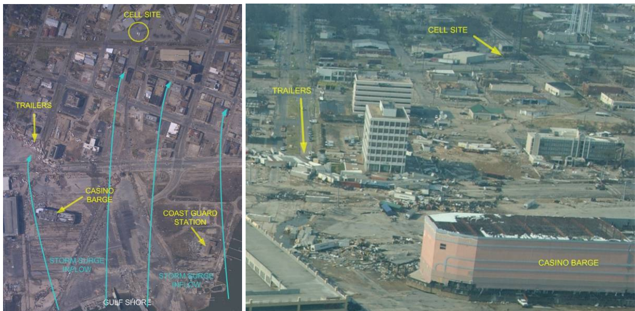
Fig. 6.36. Views of the destruction of Gulfport, Left: [6] Right: [7]
