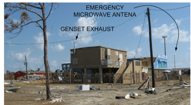
Fig. 8. A small switch facility near Crystal Beach after Hurricane Ike.
