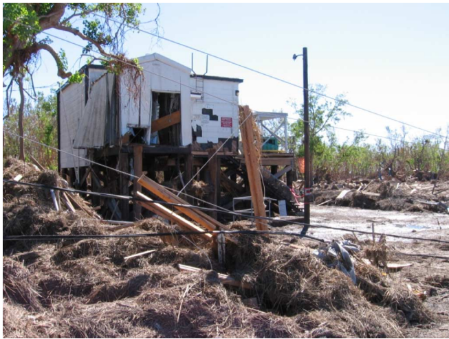
Fig. 7. Delacroix central office.
