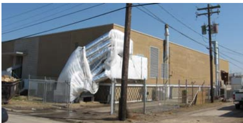
Fig. 1. AT&T's Sherwood central office in Galveston Island, Texas.
