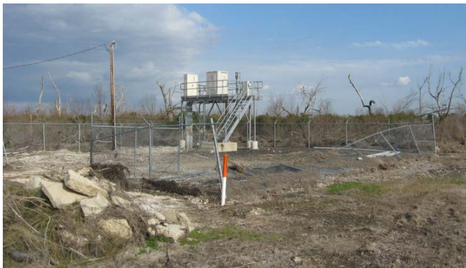
Fig. 11. A damaged fence near the DLC that replaced Delacroix Central Office, destroyed by Hurricane Katrina in 2005.
