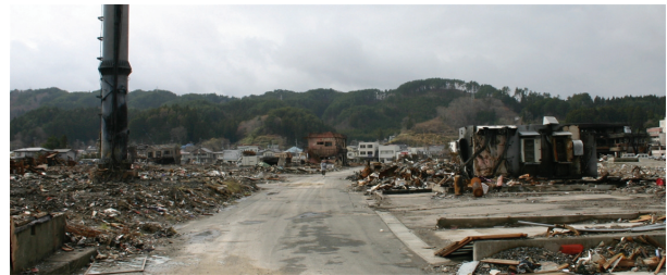
Figure 4. A cell site affected by the tsunami and fires in Yamada.
