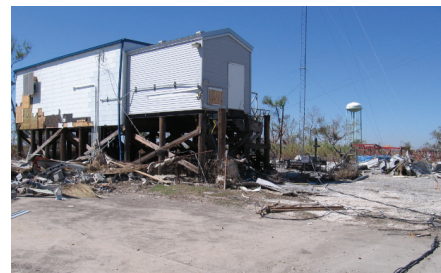
Fig. 1. Yscloskey CO after Hurricane Katrina.
