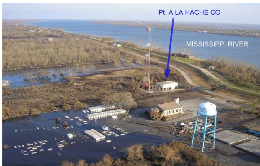
Fig. 5.42. Aerial view of Point A La Hache CO [20]
