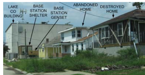
Figure 3 Homes behind AT&T's Lake CO in New Orleans.
