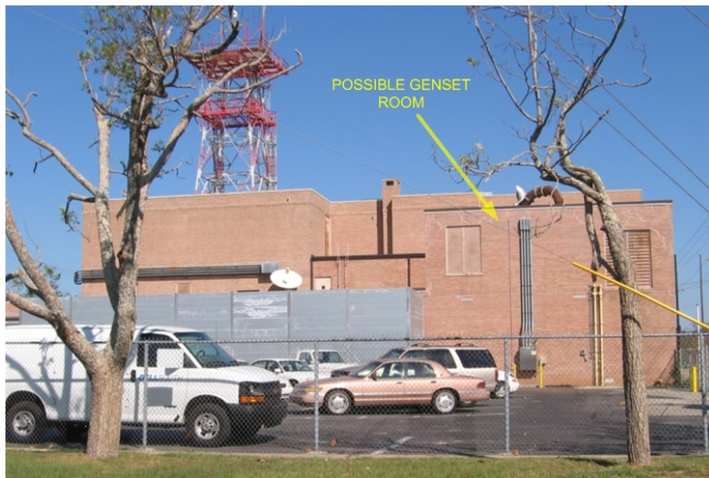
Fig. 5.21. BellSouth Gulfport CO
