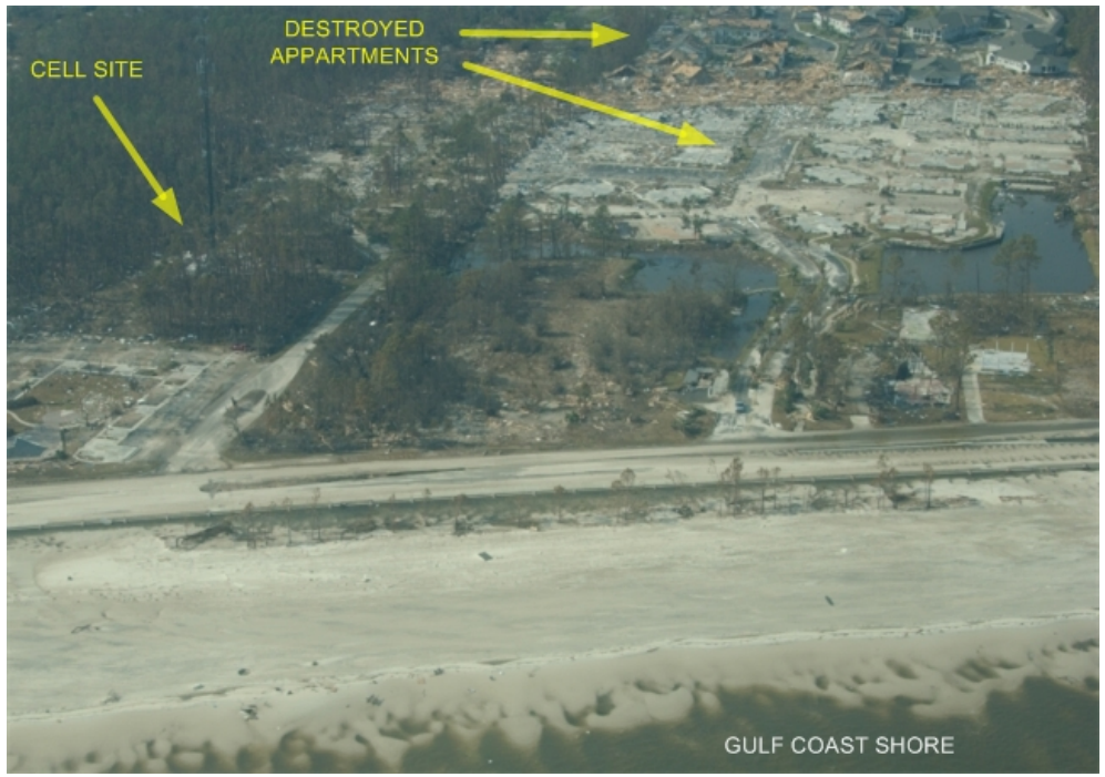
Fig. 6.18. Aerial picture showing the destruction of a cell site in Long Beach, MS [7]
