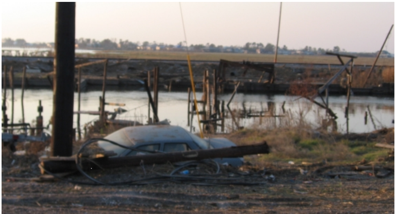
Fig. 3.19. Broken pole and remains of telephone distribution cable in Slidell, LA
