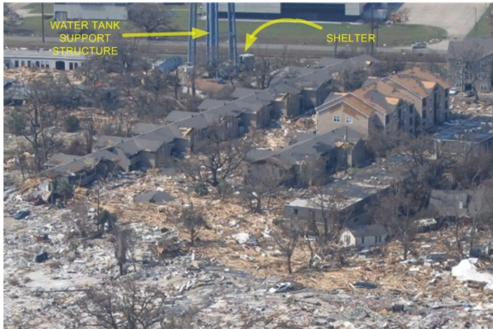
Fig. 6.22. Damage next to water tower cell site [9]
