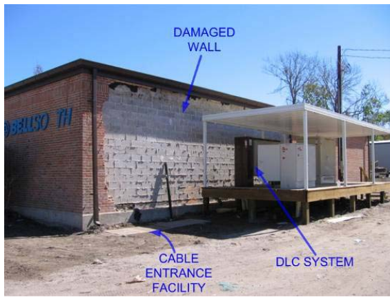
Fig. 7. Pass Christian CO showing the DLC system used to replace the destroyed switch.
