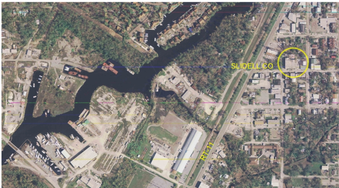
Fig. 5.20. Aerial view of Slidell CO [10]
