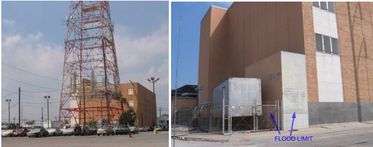
Fig. 5.58. Broadmoor CO, Left: Front, Right: Back
