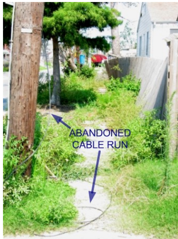
Fig. 10.1 Abandoned cable run and residence damage in an alley a few blocks east of the 17 th Street Canal, Orleans Parish, July 2006. Photo courtesy of D. Dickey.
