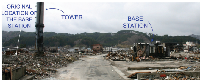
Fig. 19 A destroyed cell site by the tsunami and fire in Yamada.
