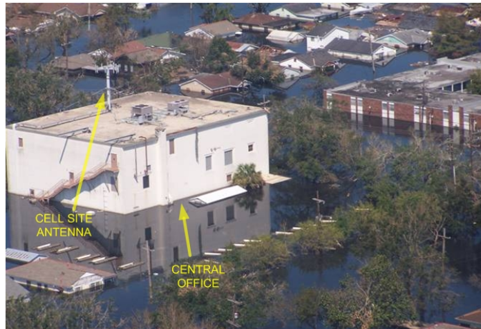
Fig. 6.49. Collocated cell site inside BellSouth Lake CO [20]
