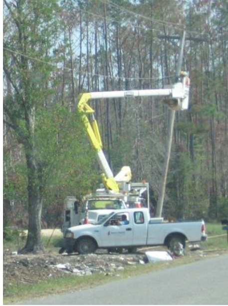
Fig. 3.12. PSTN outside plant being repaired
