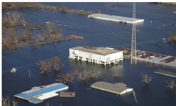
Fig. 5.60. Aerial view of Venice CO [20]
