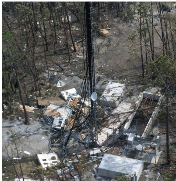
Fig. 6.17. Remains of a cell site in Long Beach, MS [36]
