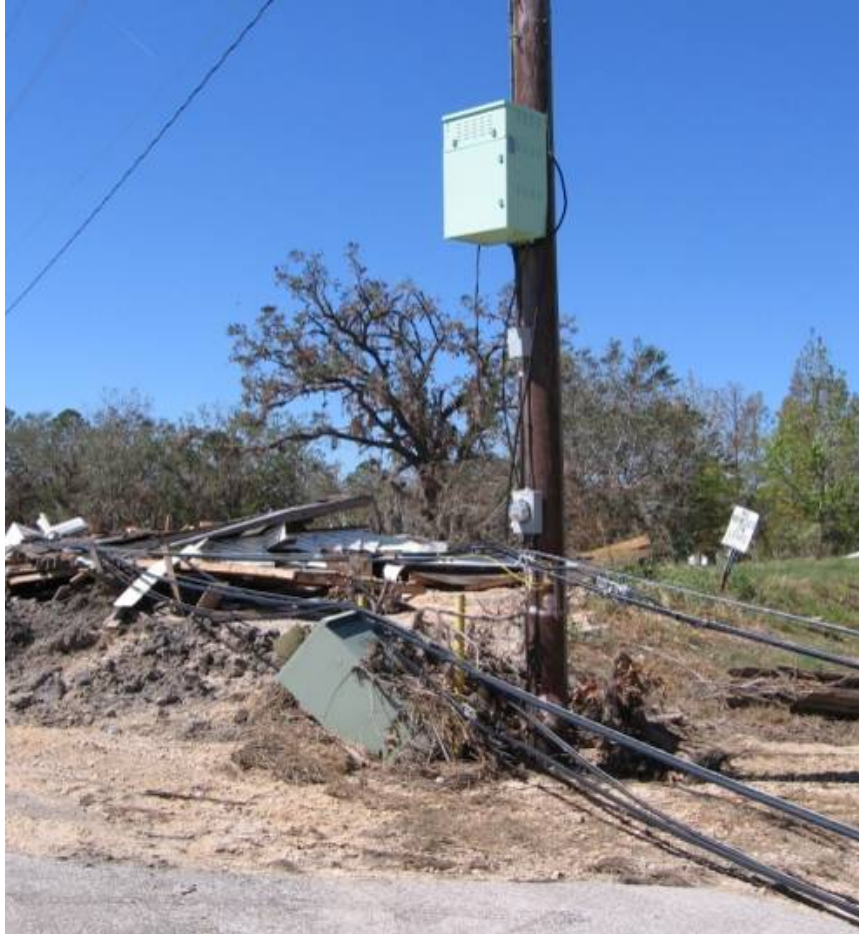
Fig. 7.11. Pole-mounted and pedestal-mounted CATV UPSs.
