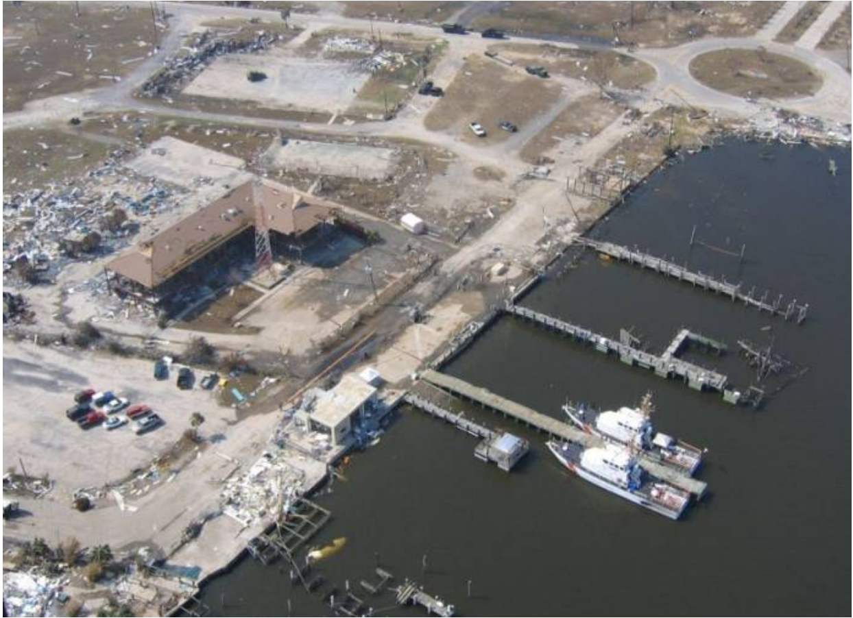
Fig. 9.3. USCG station in Gulfport, MS [9]
