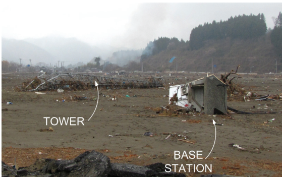
Fig. 17. A destroyed cell site near Rikuzentata.
