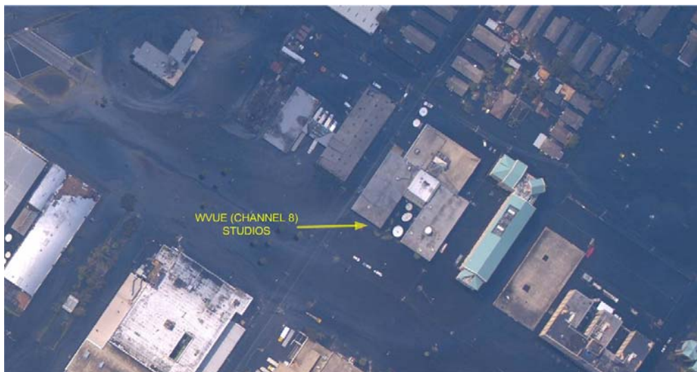
Fig. 7.5. Aerial picture of WVUE-TV studios in New Orleans, August 31 st [6]
