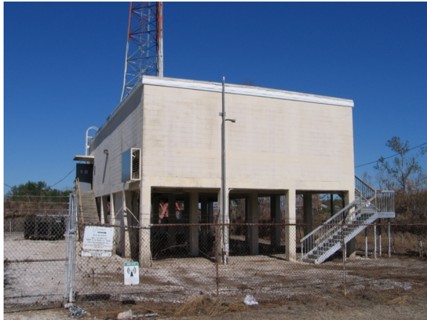
Fig. 5.41. Point A La Hache CO, October 18, 2005
