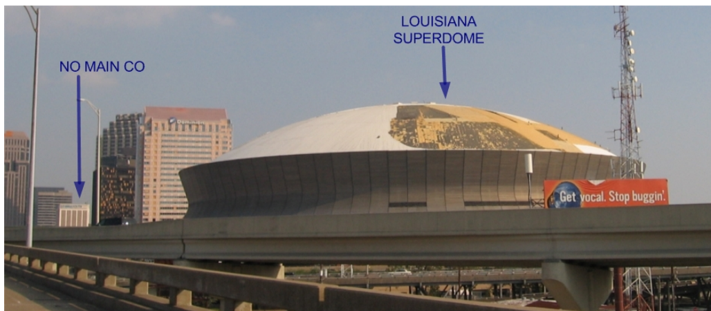
Fig. 5.13. Louisiana Superdome and the New Orleans Main CO
