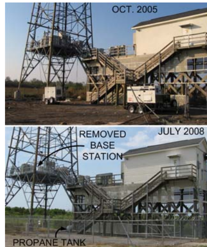
Figure 16 A closer view of the cell site in Fig. 6.
