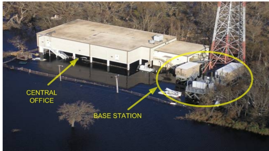
Fig. 6.14. BellSouth Buras CO showing the collocated cell site [20]
