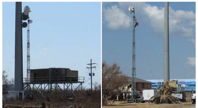
Fig. 4. South side (left) and North side (right) of an emergency microwave link in the Bolivar Peninsula.
