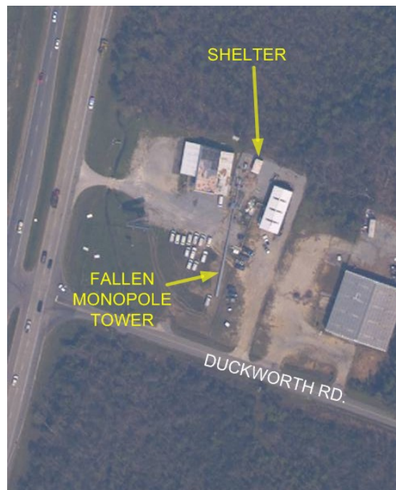
Fig. 6.68. Aerial picture of a fallen monopole tower north of Gulfport, MS [6]
