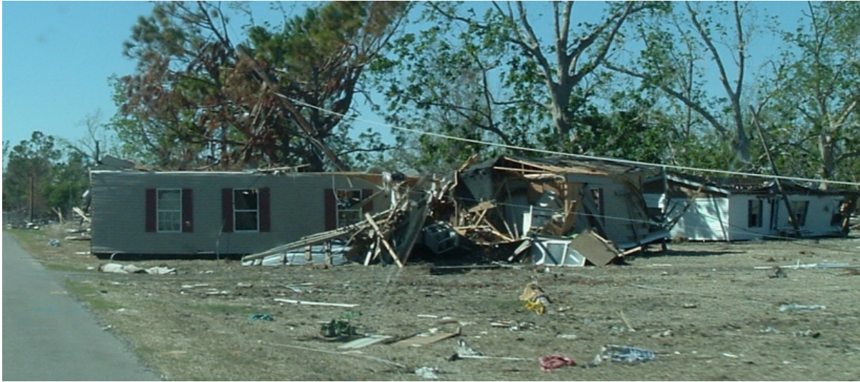
Fig. 3.4. Total destruction on Highway 15, LA
