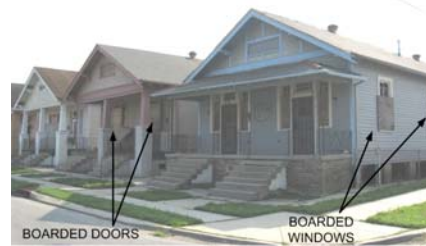
Figure 2 Mostly abandoned houses in New Orleans.
