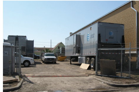
Fig. 7. Emergency mobile switches outside Sherwood CO after Hurricane Ike.
