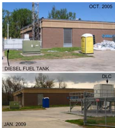
Figure 7 Former Bellsouth's St. Bernard Central Office.
