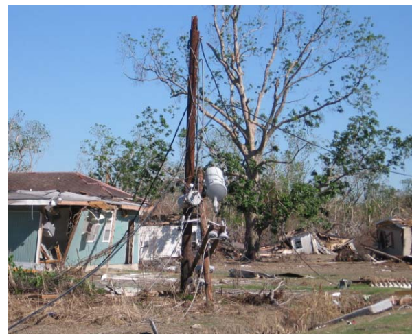
Fig. 3. Typical damage to the electric distribution grid near Pt. A La Hache, LA.
