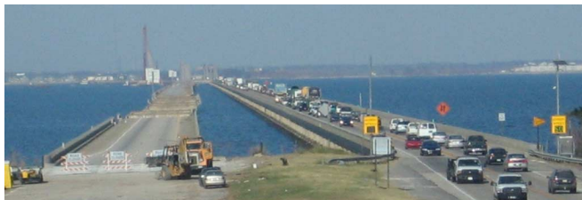
Fig. 17. I-10 bridge damage over Lake Pontchartrain.
