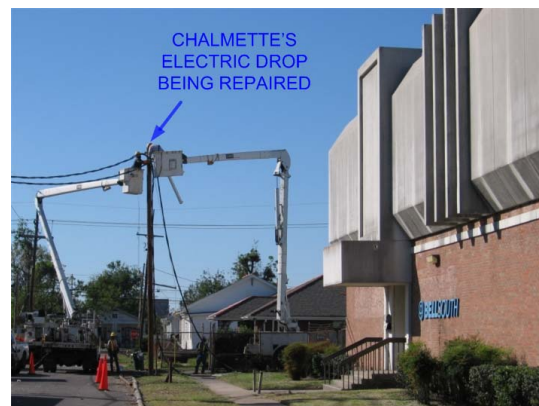
Fig. 10. Chalmette’s CO electric drop being repaired. Photo taken on October 18 th , 2006.
