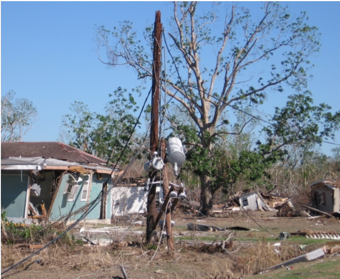
Fig. 3.3. Severe structural damage to houses and a broken pole with distribution transformer and telecom outside plant cables in Point A La Hache, LA
