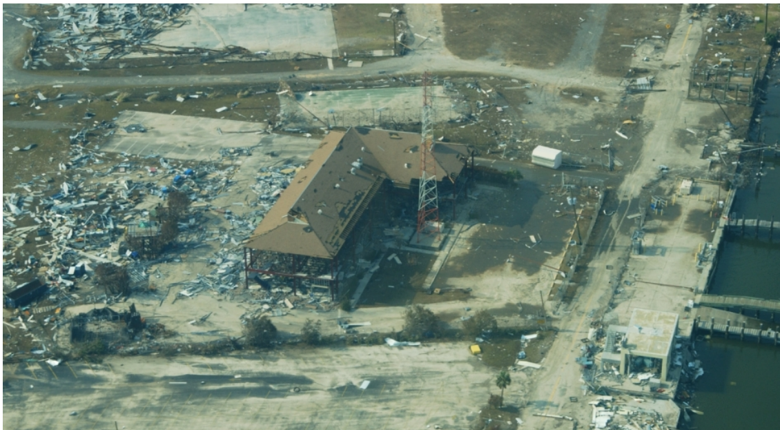
Fig. 9.2. USCG station in Gulfport, MS [7]
