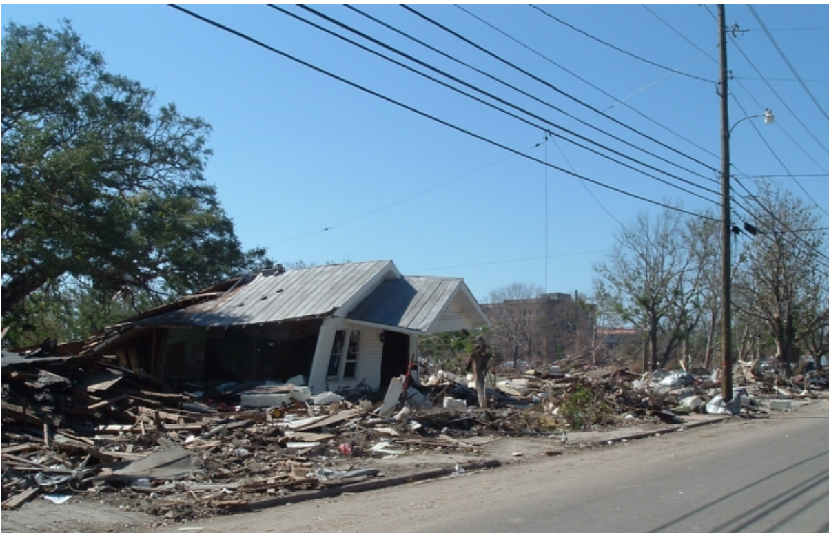
Fig. 3.7. Severe residential damage; none to electrical and PSTN distribution cables in Biloxi, MS
