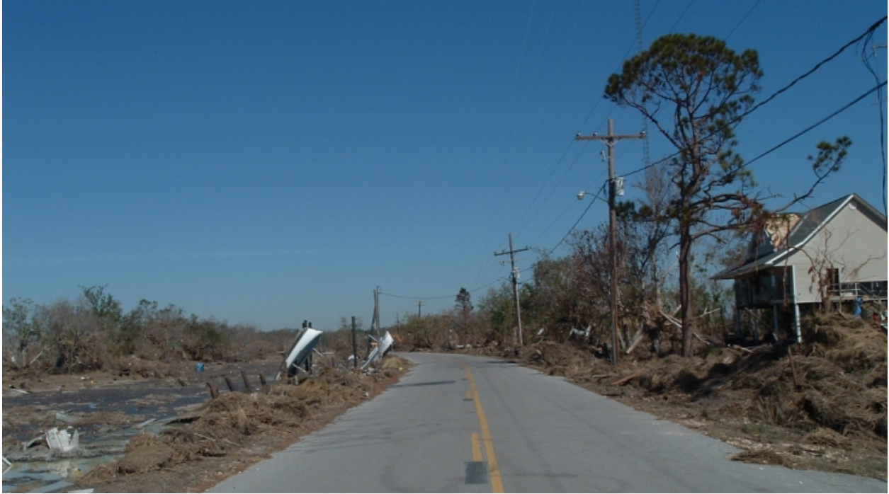
Fig. 3.10. Severe damage to construction but light damage to electrical and communication networks in Delacroix
