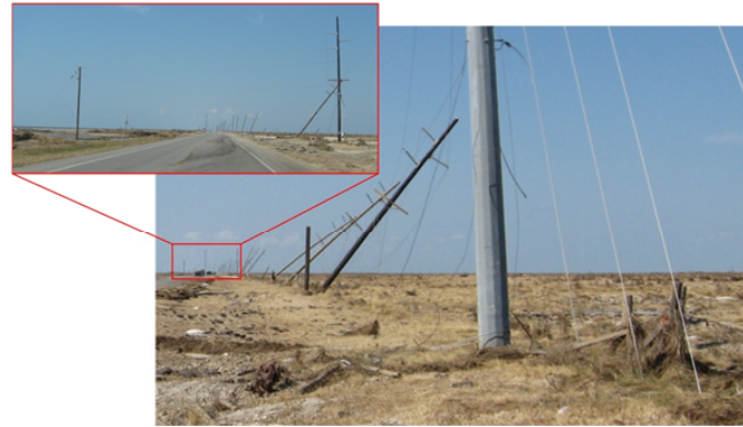
Infrastructure hardening option: Gullied poles
