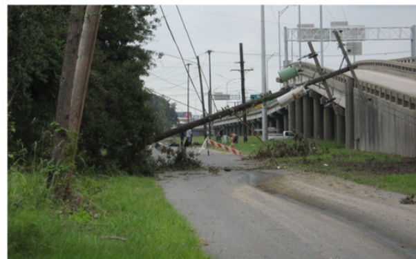
Damage caused by Gustav
