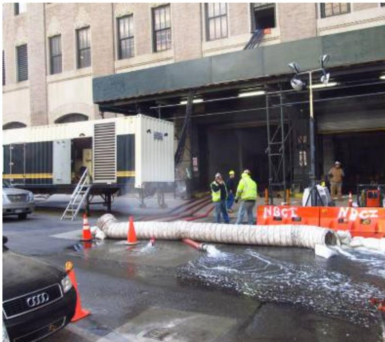
Fig. 3. Water being pumped out and a diesel generator running at the entrance on Barclay Street for Verizon's main central office in Manhattan.
