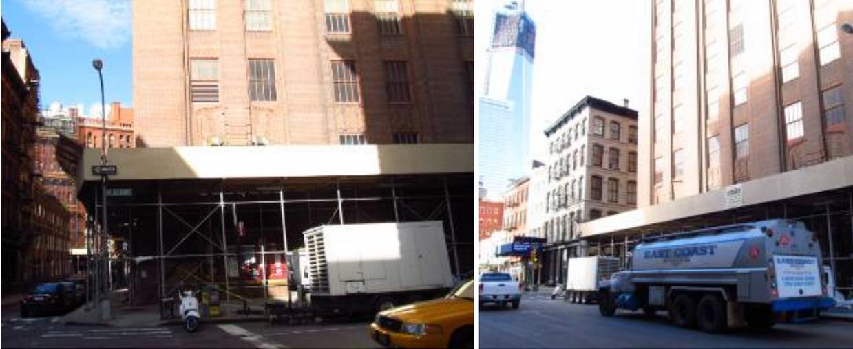
Fig. 31. Two views of the 60 Hudson Street data center showing additional small gensets in the area and a truck with diesel to replenish the fuel tanks at this site.
