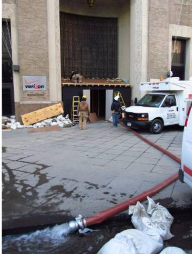
Fig. 2. Water being pump out through the main entrance of Verizon's central office at 140 West Street.
