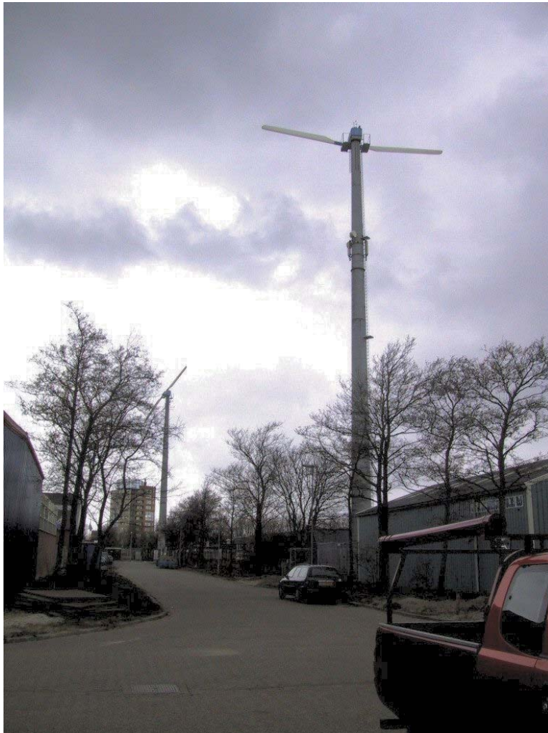
Figure 4.3: Photo of the two wind turbines at “Ambachtsweg”.
