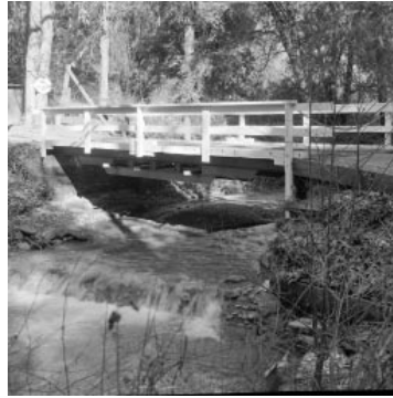
(a) Original bridge image.
