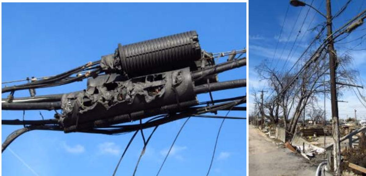
Fig. 33. Damage from a fire affecting communications infrastructure.
