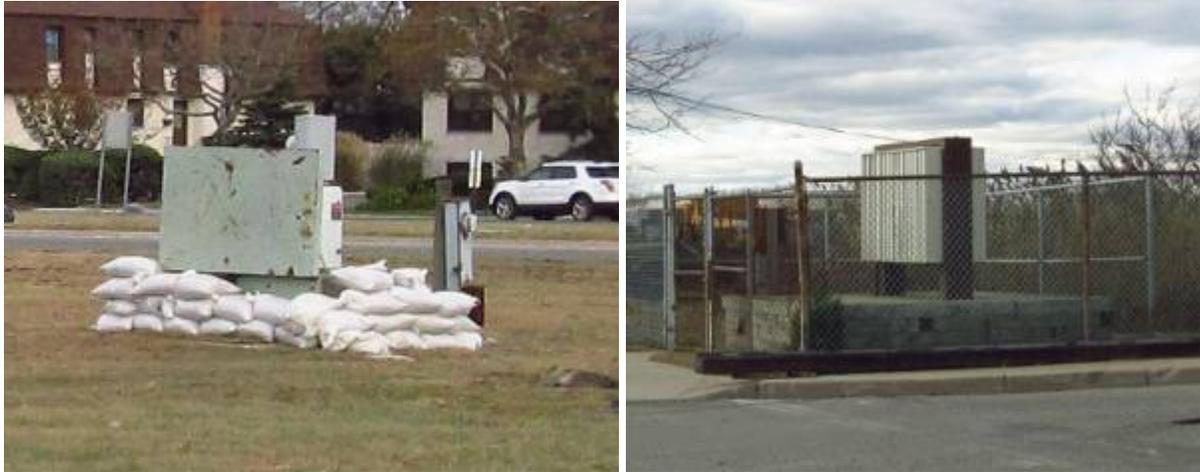
Fig. 32. A vault (left) and a DLC RT cabinet (right) in the Rockaway Peninsula.
