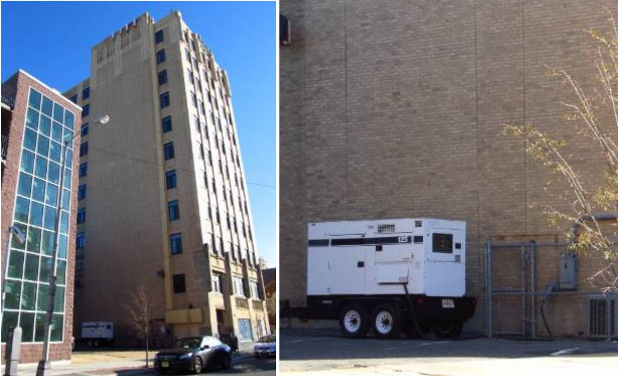
Fig. 18 A rooftop cell site in Ausbury Park powered by a genset at street level. Notice the standard connector for the genset.
