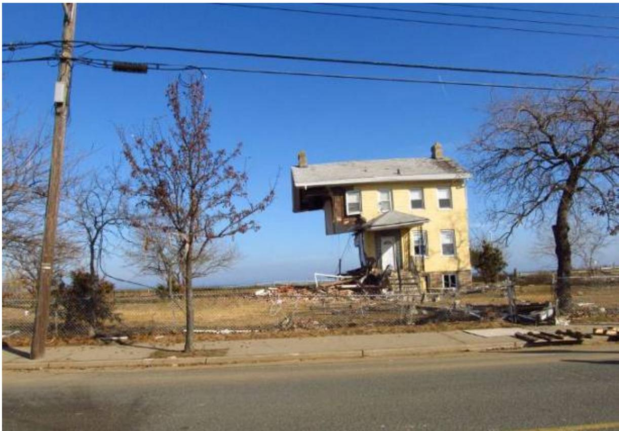
Fig. 38. Important damage to dwellings in Union Beach but little damage to poles.
