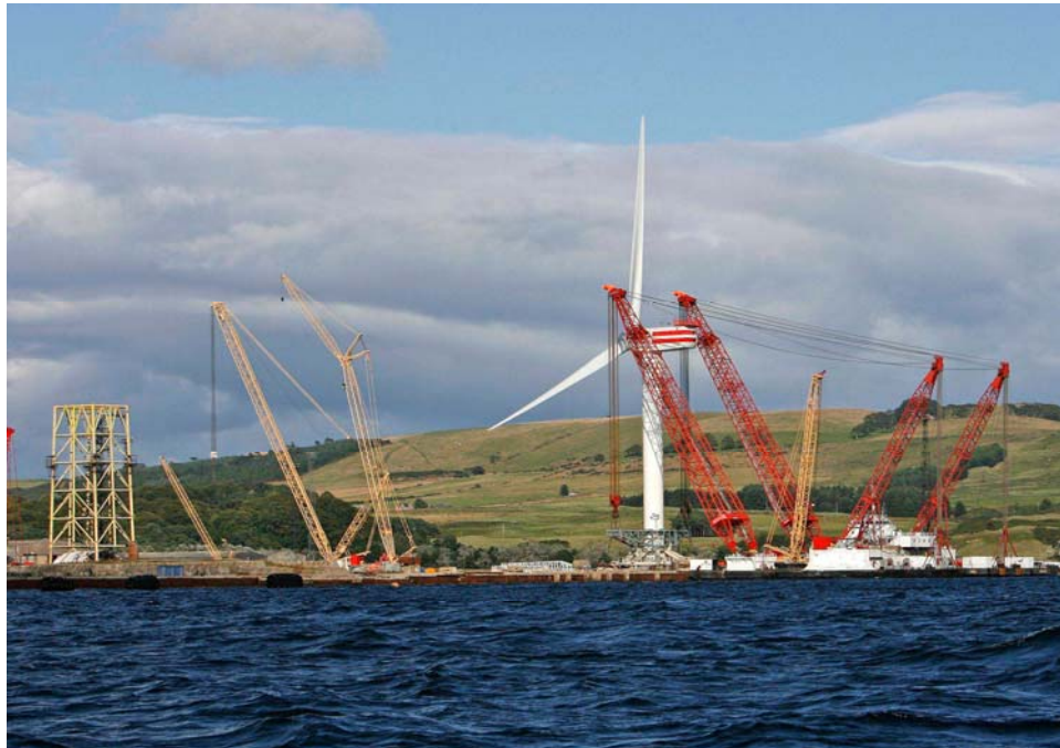
Plate 1. Offshore Wind Turbine Construction
